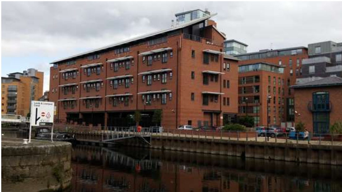
Figure 14. The Fearn's Wharf building, built on a raised platform to adapt to floods
