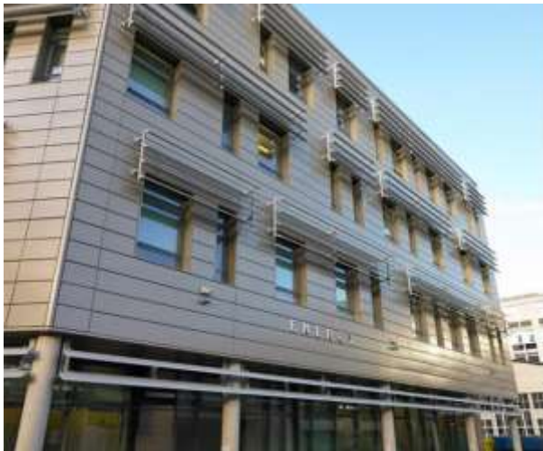
Figure 7. Solar shading devices on the Energy Research building at University of Leeds
