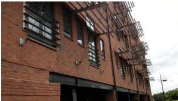
Figure 5. Solar shading devices on the Fearn's Wharf building.
