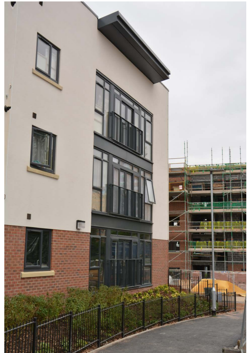
Building new homes in Leeds
