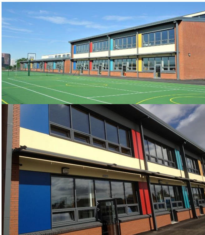
Designed by _space group and (the former) Education Leeds, with Interserve Project Services
